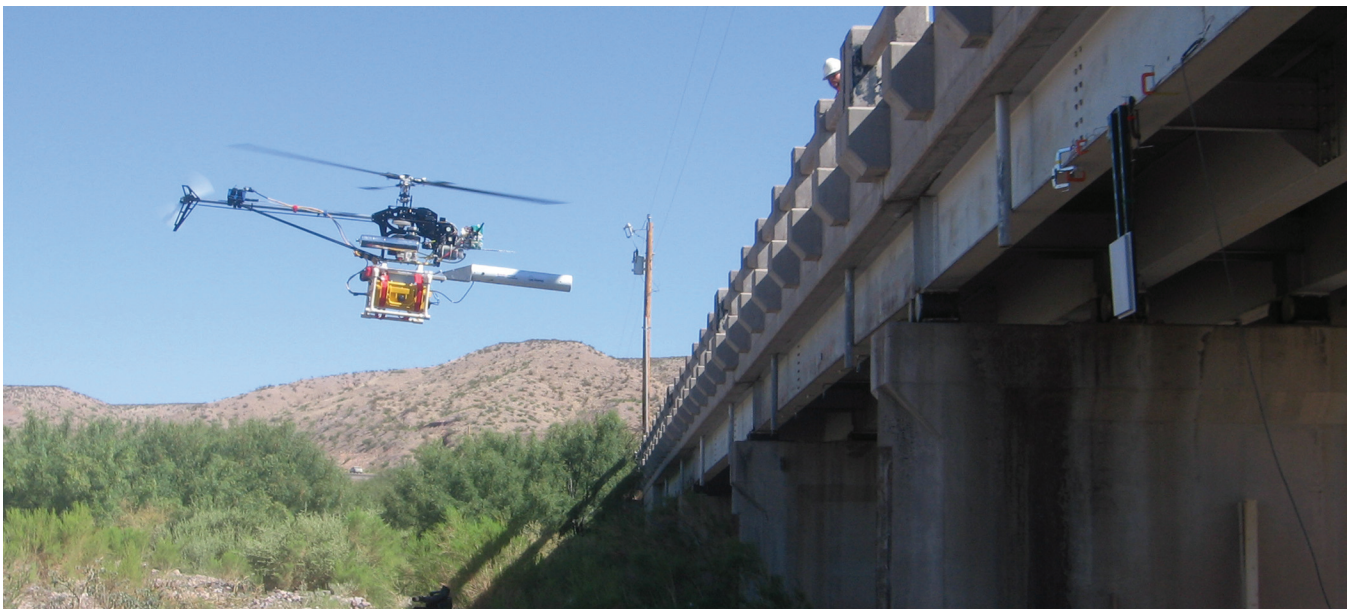
The helicopter delivers power to the sensor nodes mounted on a bridge structure.
