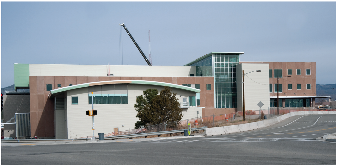
The Radiological Laboratory/Utility/Office Building will house office and light laboratory space and is the first phase of the CMRR Project. LANL will conduct very small-scale plutonium analysis, limiting the total amount of plutonium in the building to less than 8.4 grams at any one time.
